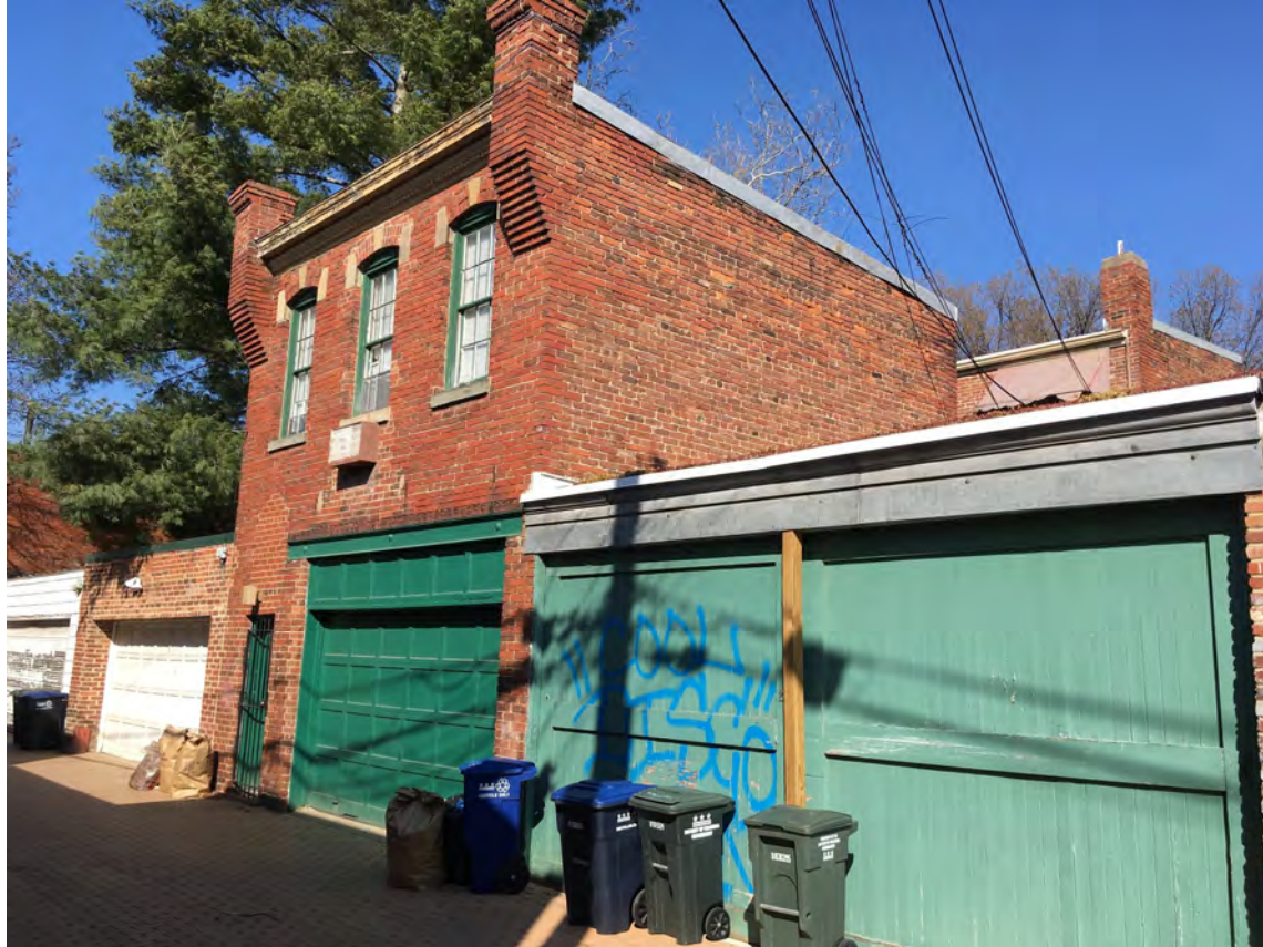
GARAGES TO THE NORTH
