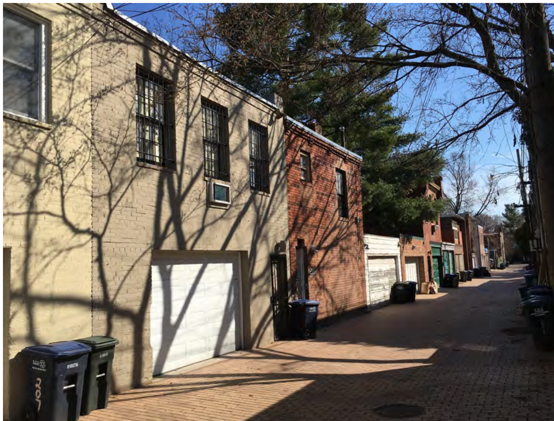
GARAGES TO THE NORTH
