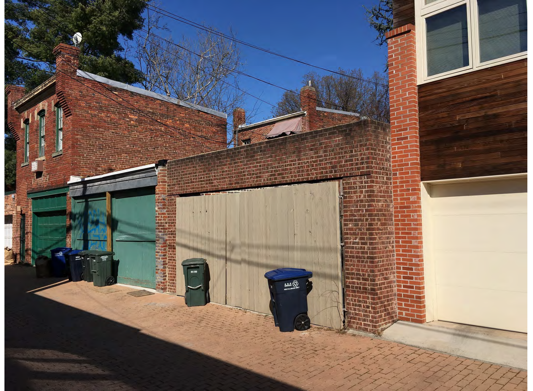
EXISTING SECURITY WALLS AND GARAGE DOOR AT 221 10 TH STREET SE
